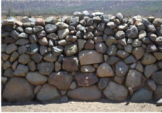
A close-up photograph of a stone wall (pirka) constructed from large, irregular stones. The stones are stacked in a regular pattern, with larger stones forming the base and smaller stones filling the upper sections. The wall is built on a dirt surface.                           | <p>Detalle de pirka en primer plano.</p>                            |
